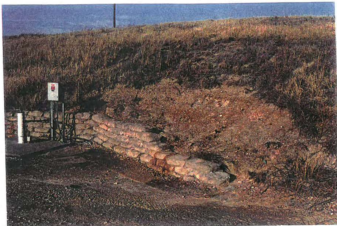
Photo No. 1: View of Travis County Landfill erosion of cover at leachate seep.
