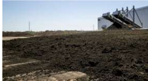
Anaerobically digested Class B biosolids at Hornsby Bend wastewater treatment plant on June 16. JAY JANNER/AMERICAN-STATESMAN
